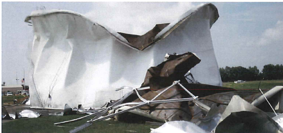
The gasoline storage tank at the TEPPCO McRae Terminal following the 2009 hot work accident that killed three workers.
